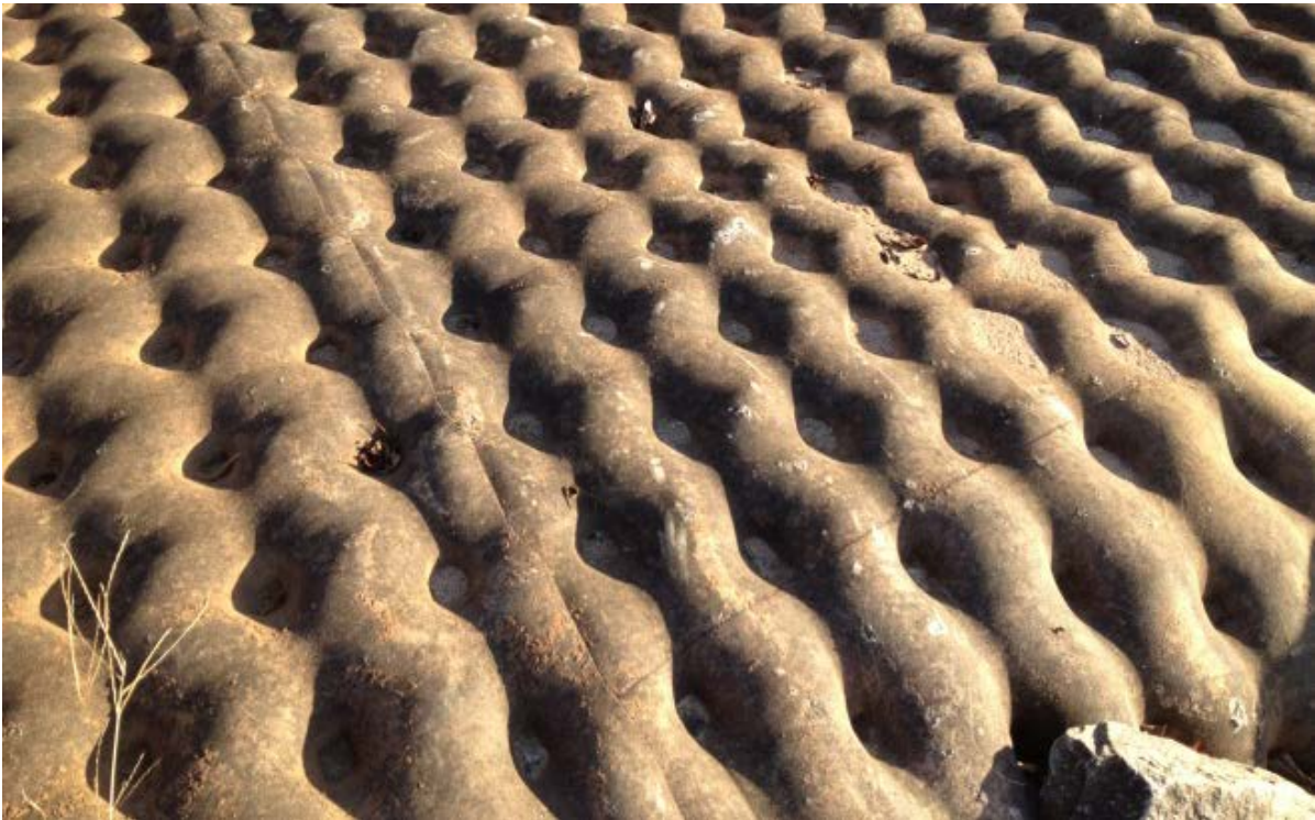
Concrete Mattress Structure Exposed
